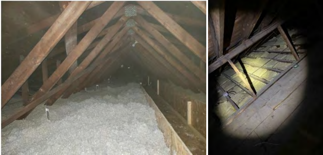
Figure 14. Examples of installed attic insulation using cellulose (left) and fiberglass (right)
