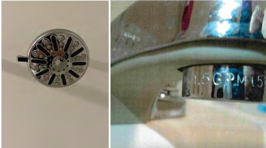
Figure 15. Example of installed low flow showerhead (left) and faucet aerator (right)
