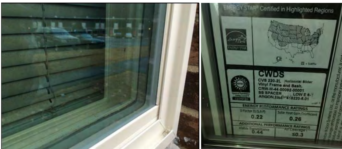
Figure 11. Example of installed window and window label
