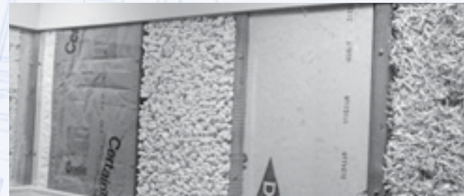
A cross section of insulation displayed in the E-House
