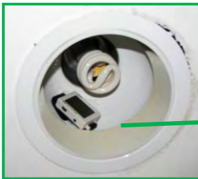
This is a curved recessed fixture – logger is installed using a 3M strip on the Velcro strap to stick to the curved surface
