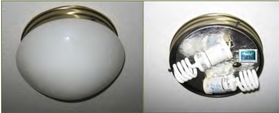
Figure 8: Dome Style Fixture – Remove Dome
