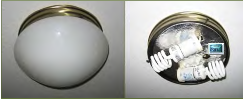
Figure 8: Flush Mount Style Fixture – Remove Dome
