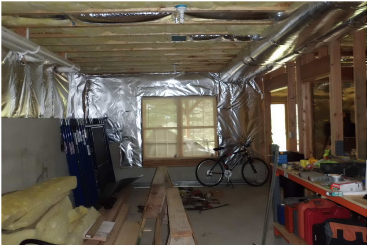
Figure 0-2: Insulated Walkout Basement Walls
