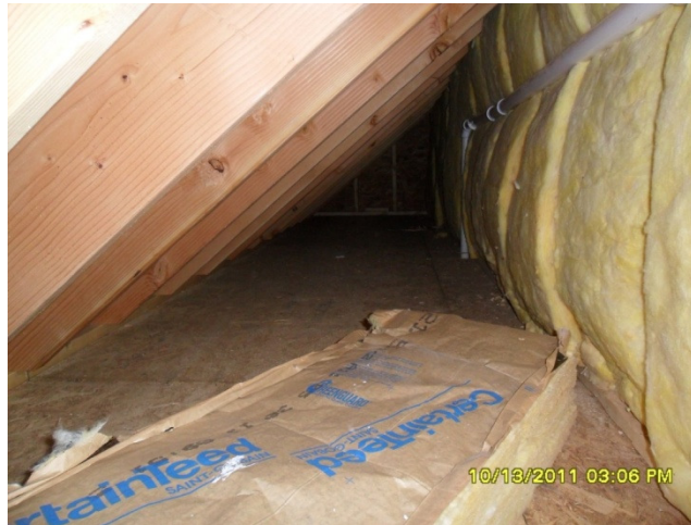
Figure 0-3: Grade III Fiberglass Batts—Attic Kneewalls
