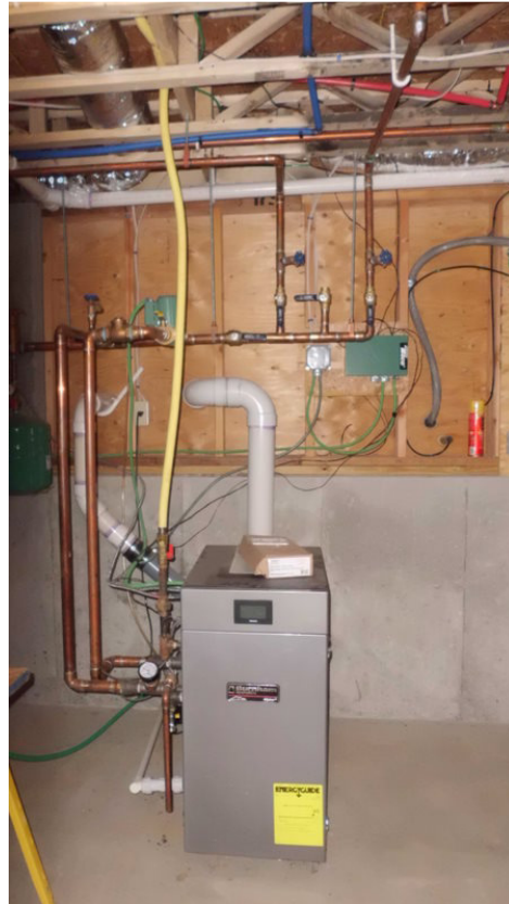
Figure 0-3: Uninsulated Above Grade Basement Walls
