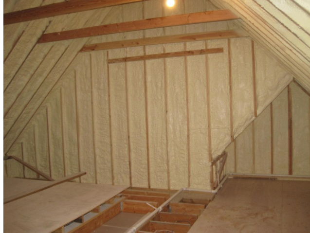
Figure 0-1: Grade I Closed Cell Spray Foam—Exterior Walls
