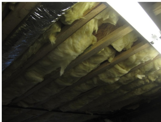
Figure 0-5: Grade III Fiberglass Batts—Frame Floor
