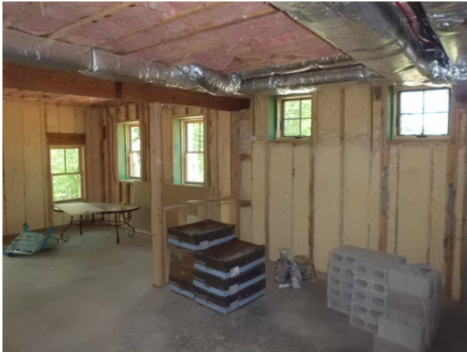
Figure 0-8: Walls with Closed Cell Spray Foam Insulation
