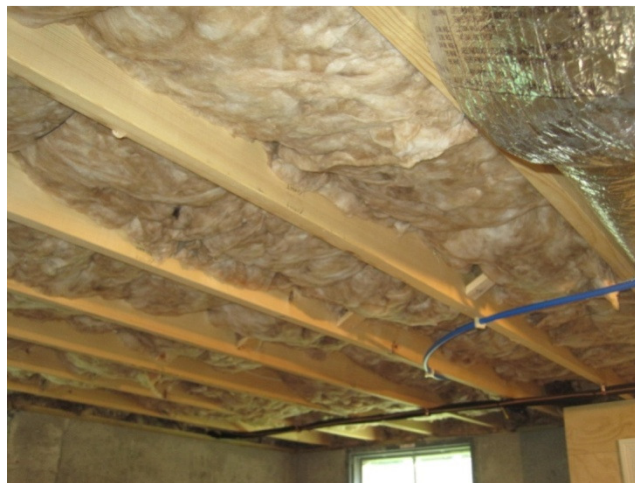
Figure 0-4: Grade II Fiberglass Batts—Frame Floor
