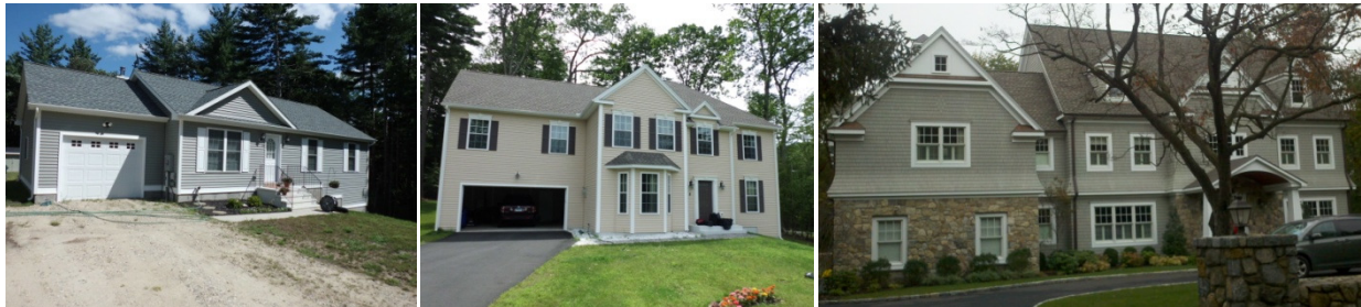
Figure 5-2: Examples of Inspected Homes
