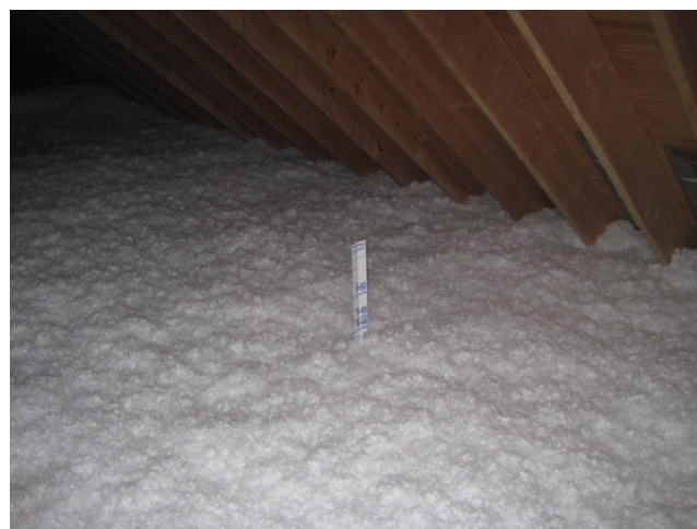
Figure 0-6: Grade I Blown Fiberglass—Attic
