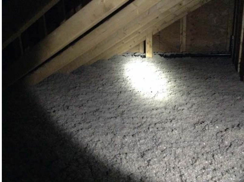
Figure 29: Grade I Blown Cellulose—Attic
