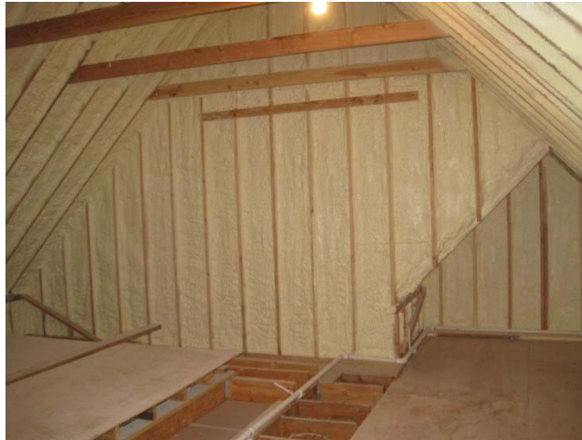
Figure 24: Grade I Closed-Cell Spray Foam—Exterior Walls
