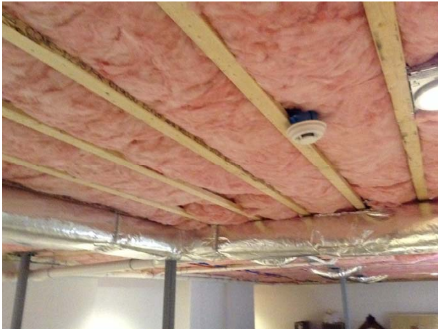
Figure 27: Grade II Fiberglass Batts—Frame Floor
