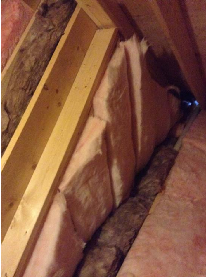
Figure 26: Grade III Fiberglass Batts—Attic Kneewalls
