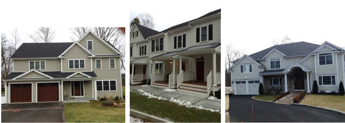
Figure 4: Examples of Inspected Homes
