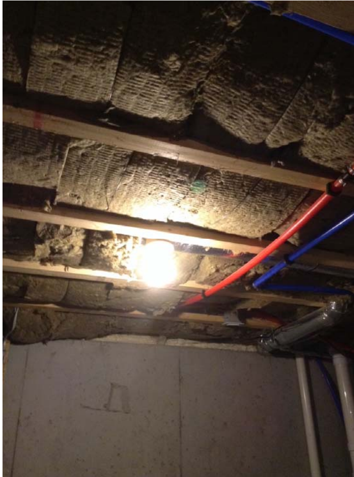
Figure 28: Grade III Fiberglass Batts—Frame Floor
