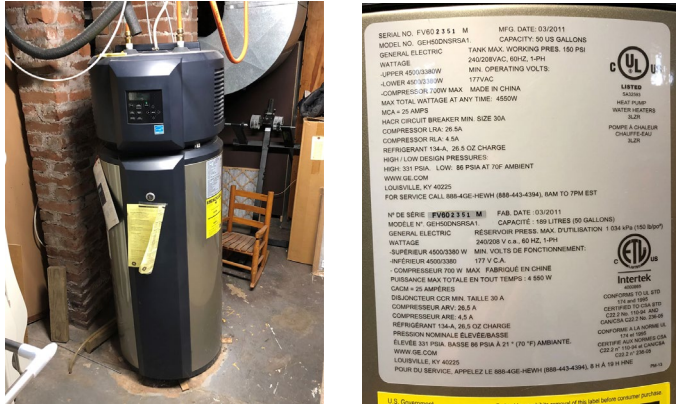
Figure 5. Example of Verification Picture Provided by Respondent
